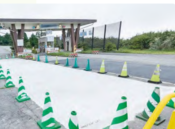
Roadway using next-generation low-carbon semi-flexible pavement
