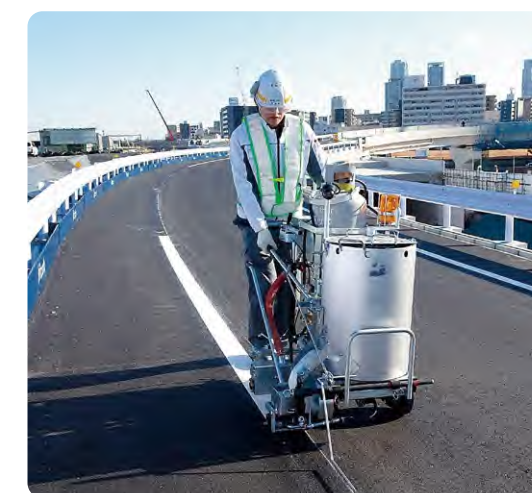
Applying road marking paint made from CO 2 recycling artificial limestone
